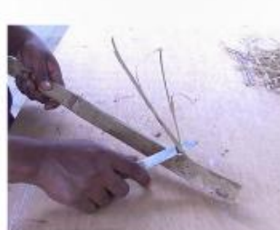
Figs 62 a 64 – Retirando os diafragmas e aparando as ripas
